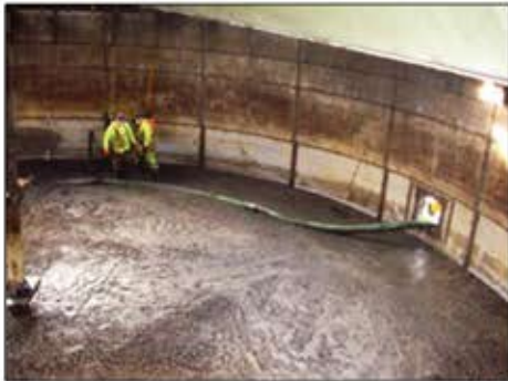
Sludge can be removed and refined to offset cleaning costs. Paraffin wax can be liquified using GP-DiSolv™ Safety Solvent.
